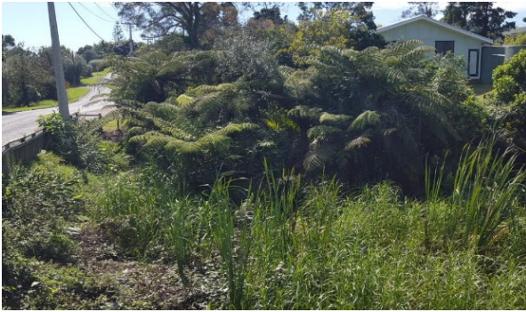
Natural wetland induced due to a culvert
