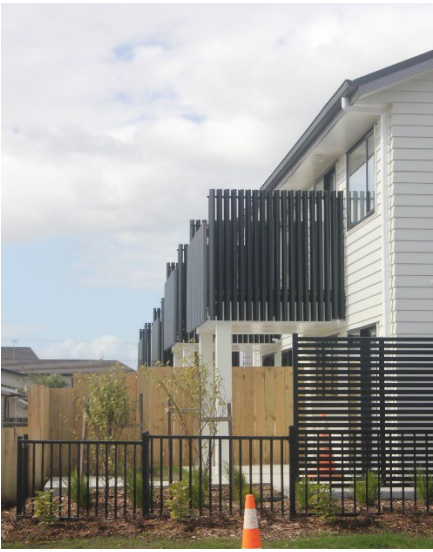
Image 7: Poor example of projecting balconies overlooking adjacent site
